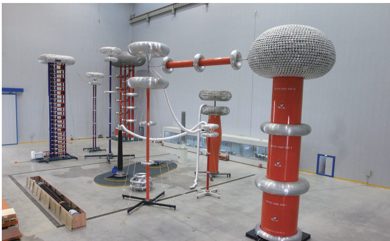
◎ 特高压试验室 Extra High Voltage Laboratory
